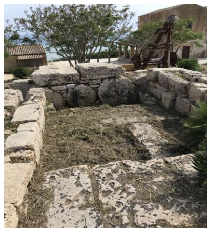
2. Tower on the South-West corner
